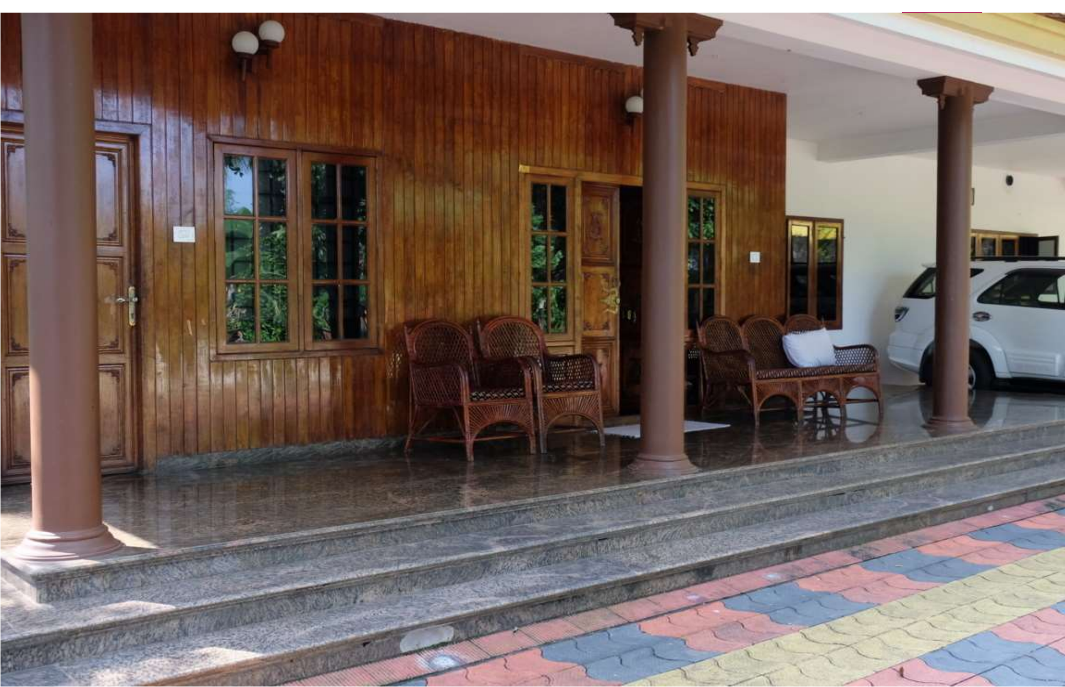
Guest House : Front view
