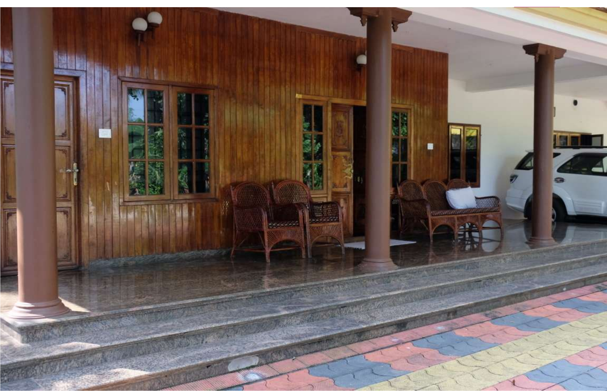
Guest House : Front view
